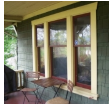
Flat board trim around perimeter of window, over siding
