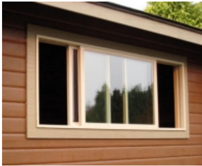
Flat board trim around perimeter of window, over siding
