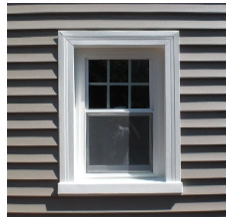
Brick-moulding overlapping siding
