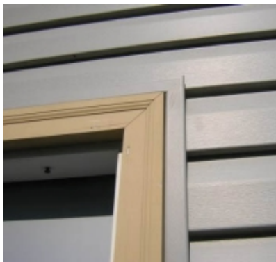
J-mould applied to siding and butted up to window
